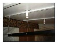
Step 2 - Turn the clip in the screen door bracket to release the bottom of the door. The clip will fit through the hole in the bracket. Lift the bottom of the door off of the rail and lower to the floor.
