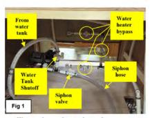
Water valves and water heater bypass
