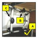
Factory installed 3-valve water heater bypass
