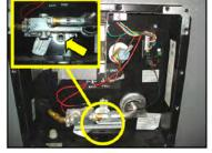
Water heater drain plug location
